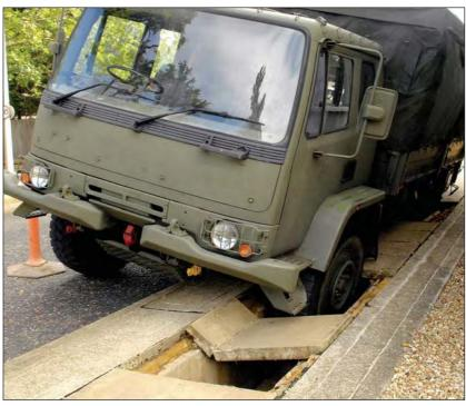
Damaged concrete trench covers in need of replacement to meet Health & Safety Regulations
